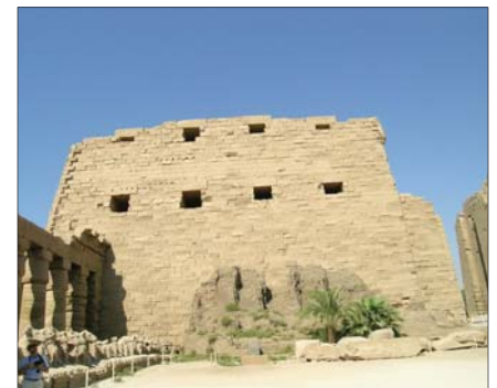
Pylon I with remnants of mud brick ramp in the Shoshenq I Court.
