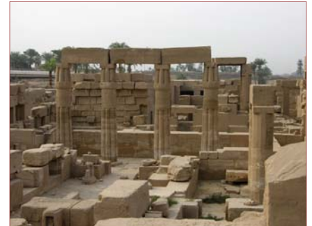
Closed papyrus form columns from the Akhmenu’s “botanical room.” On the right are an example of fluted/fasciculated columns.
