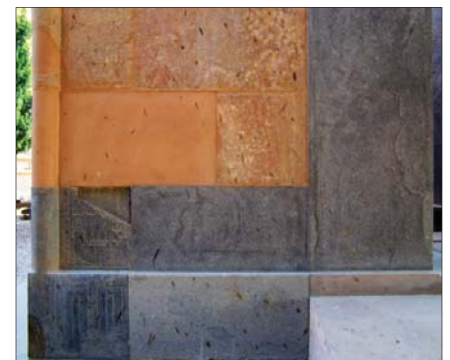
Red quartzite was used to construct the “red chapel” of Hatshepsut. Black granite was used for the doorways and the base.
