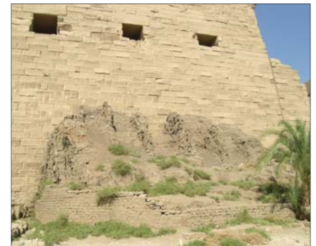
The mud brick ramp used in the construction of pylon I can still be seen today.
